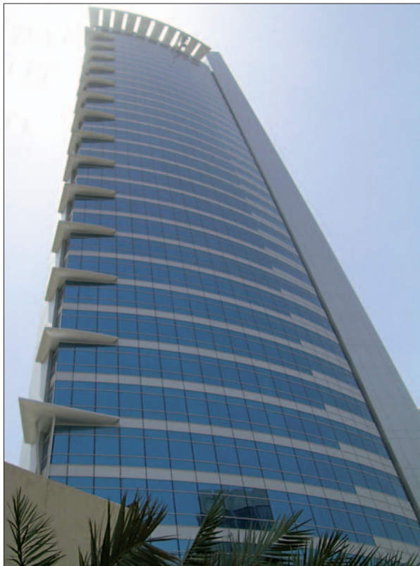
Arec Headquarter Building "Kuwait City"
